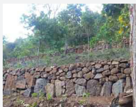
Stone bunding at Tumkur of B.Kalakote GP
